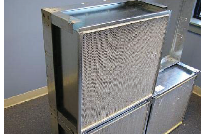
Figure 101: Filter Placed Inside of Frame
