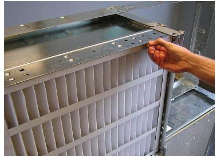
Figure 111: Installation of Prefilter Into Frame
