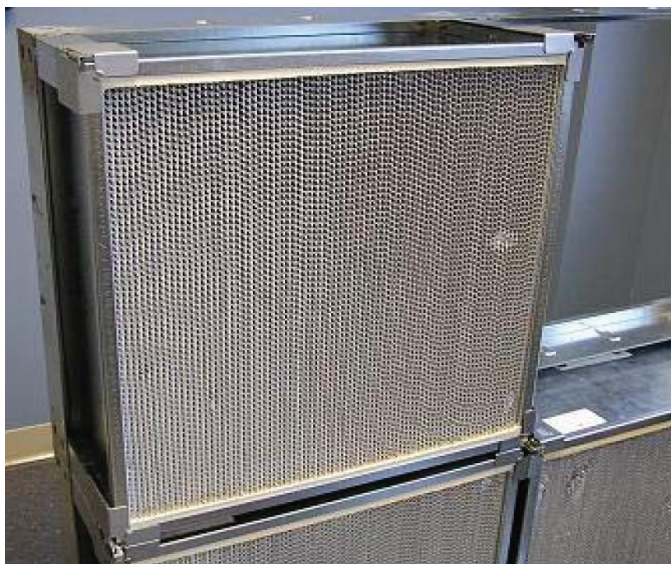
Figure 105: Properly Installed Filter Inside of the Frame
